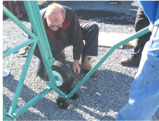
Fig. 18. Using Lifter bar, install the Wheels on both sides of A-Frame as shown. **This is a 2-Person operation!** Attempting this by yourself can put you off-balance, exposing you to serious injury or a fall ,especially when removing Wheels at the Roof Edge.
