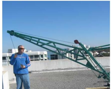
Figs 12 –16. Lift back end of Hoist and install Swing Arm into Pivot Bearings. Applying grease to Pins on Swing Arm will make this step easier. Locate Winch Unit on ground in a nearby position. Hook Power Unit up to Winch Unit and unwind enough Cable to install Mast Pulley at the top of A-frame and route Cable through the Sheave at the end of Swing Arm. Lower back end of Hoist down to roof.
